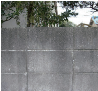
Before/洗浄後施工
